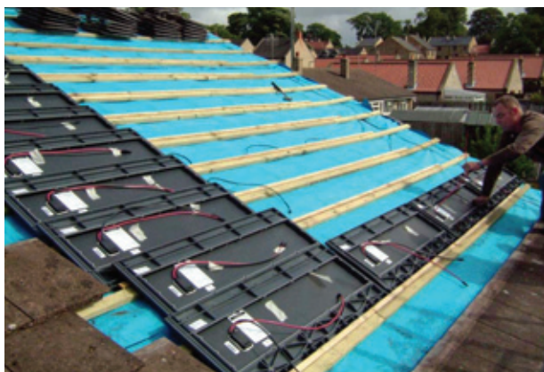
Installation of photo-voltaic roofing tiles to a rural property.
