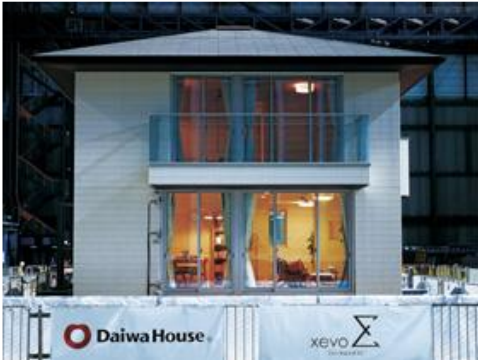
Consecutive full-scale earthquake simulation testing of the xevo \Sigma at E-Defense
