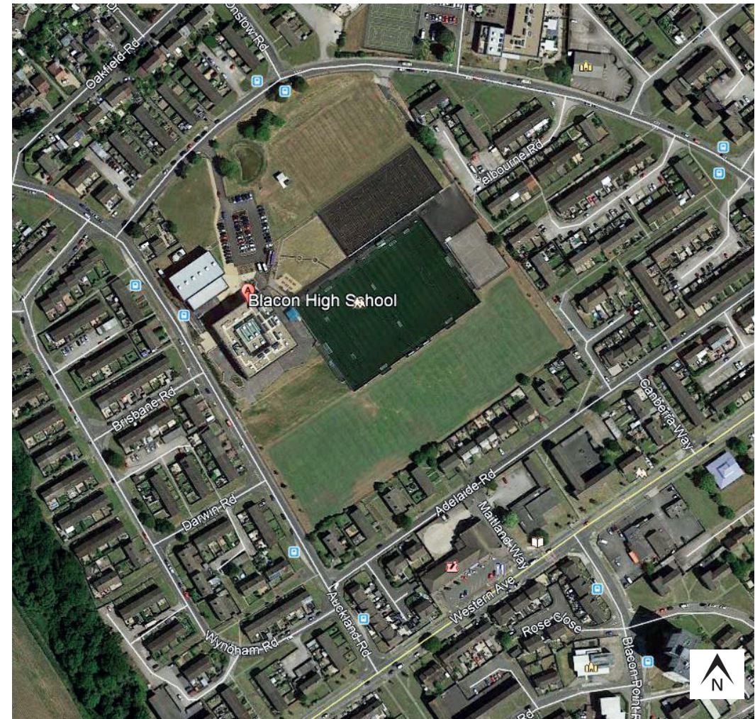
Aerial shot showing the current Blacon High School Source: Google Earth. Image date: 25 June 2018
